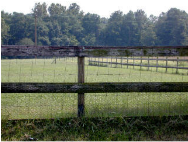
Board fence with wire mesh
