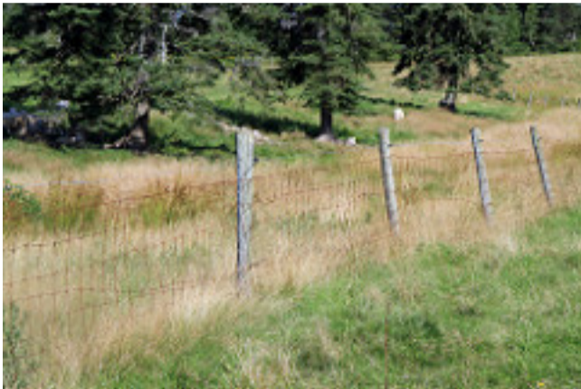
Fence in disrepair
